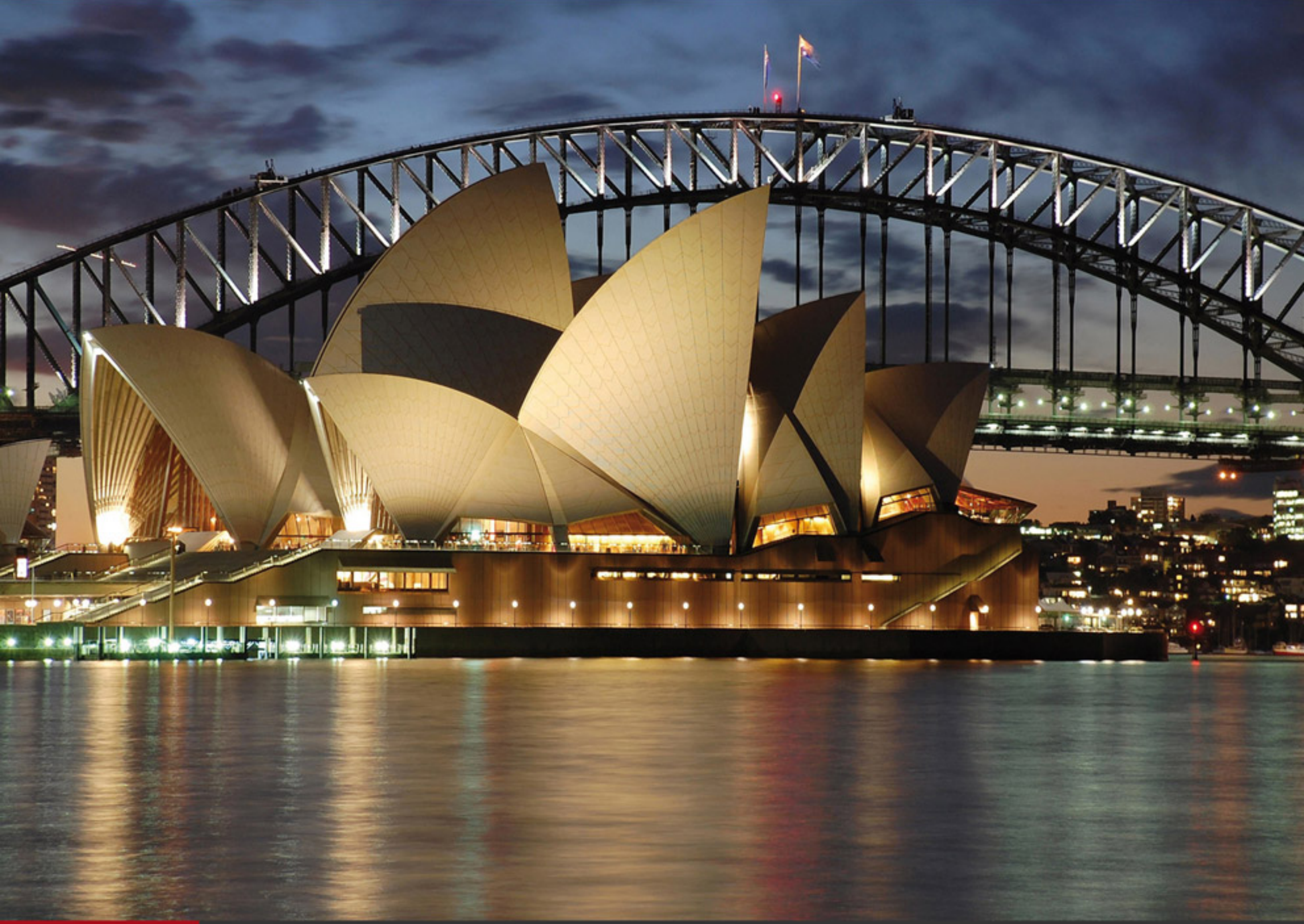
Opera Building / Sydney
